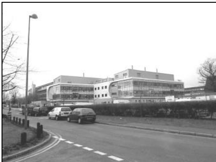
View from the East Car Park, 19 January 2004
